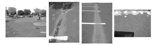
As can be seen, the appearance of the seal coated roads began deteriorating within the first year; tire marks became clearly visible and repairs were still very visible under the seal coat.
